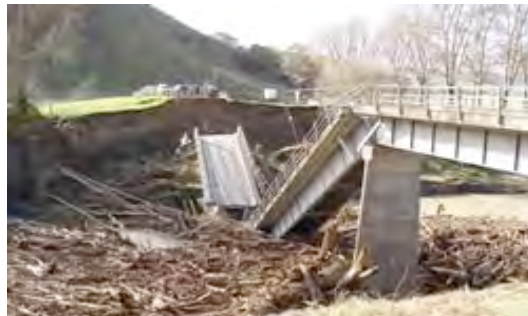
This bridge in Mangamahu shows the destruction, 2004.
