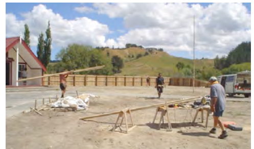
Constructions at Kauangaroa Marae.
