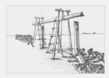
Figure 2: Hoisting the tāhuhu (Treadwell, 2014, p. 98, image used with permission)
